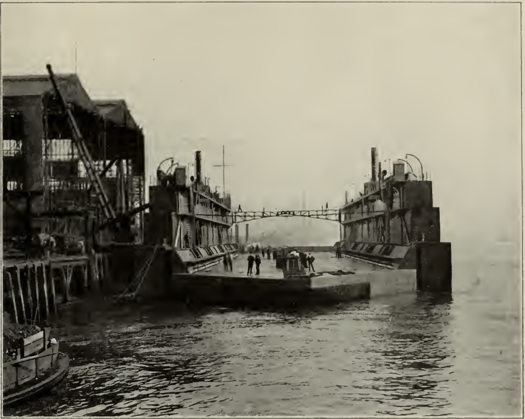
THE DURBAN FLOATING DOCK AT THE BUILDERS' WORKS.
